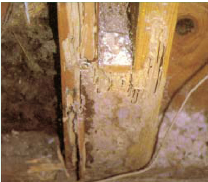
Figure 8. Formosan termite-produced carton nest in a structure.
