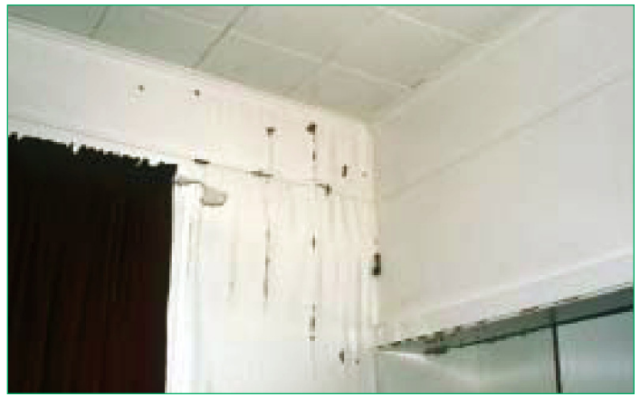
Figure 12. Shelter tubes on interior walls.
